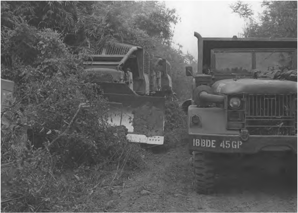
A dump truck and Rome plow begin clearing and widening Highway 9 during the opening phase of LAM SON 719.
